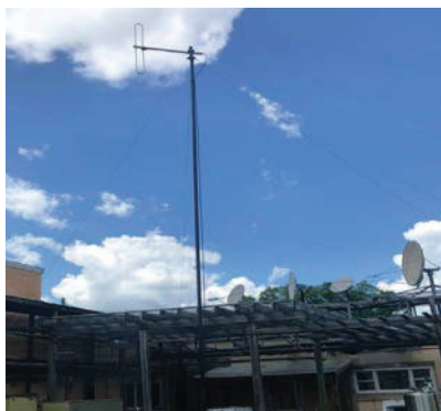
Above: Portable emergency transmitter mast and antenna being tested at WCVE-FM, Richmond, VA
